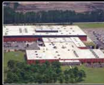
CONWAY, SC Steel Foundry and Manufacturing Plant
